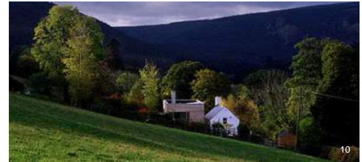
Contemporary extension to rural cottage adapting site contours into the design.
